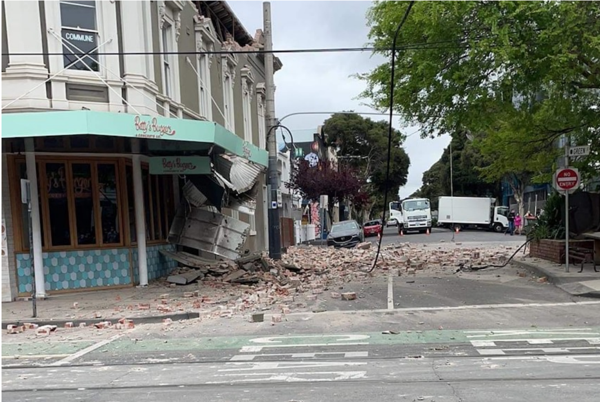
Damaged building on Chapel Street (Photo from ABC News)
